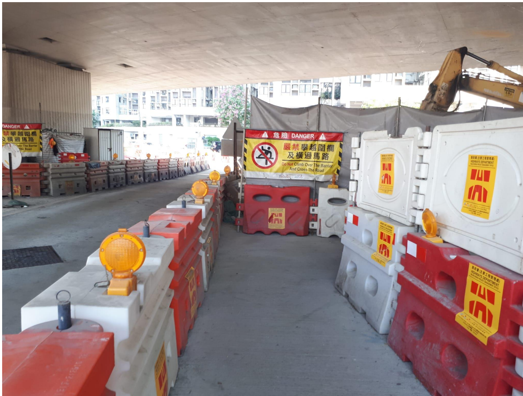
Remark 2: Photo record of on-site inspection
