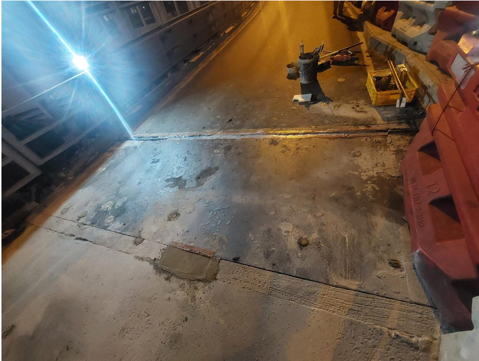
Remark 2: Photo record of rectification works
